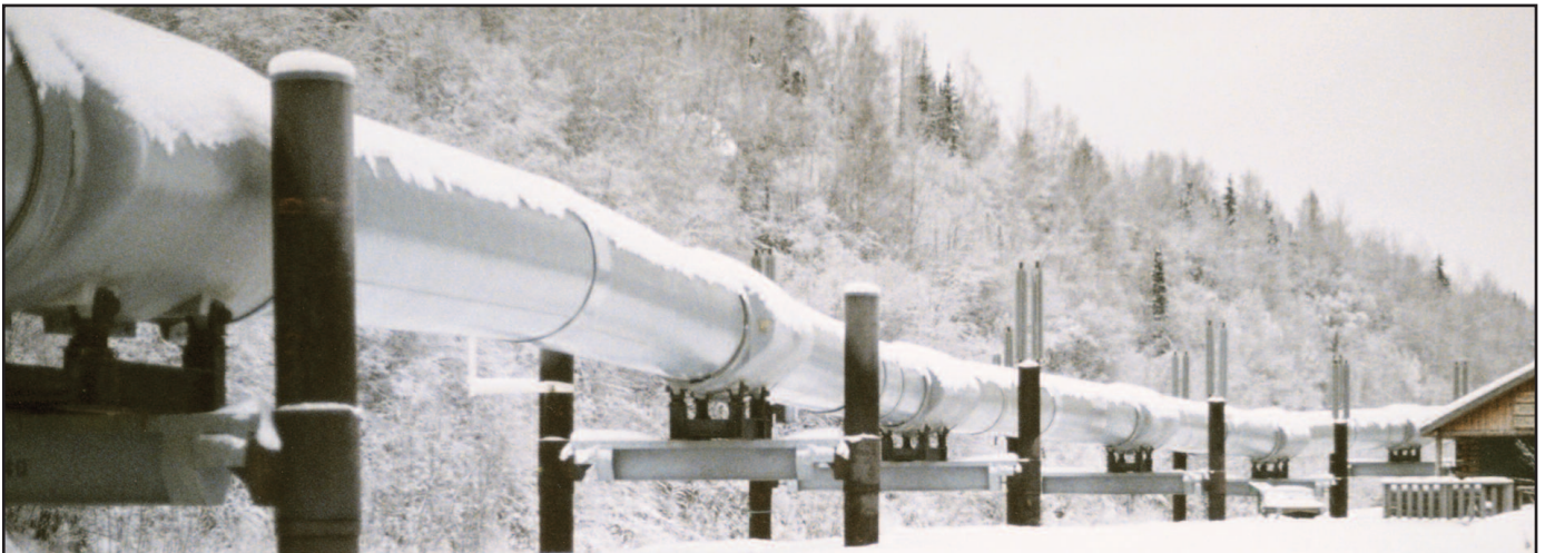
The 800 mile long 48 inch diameter Trans Alaska Pipeline System was constructed using Lincoln Electric Pipeliners® welders.
